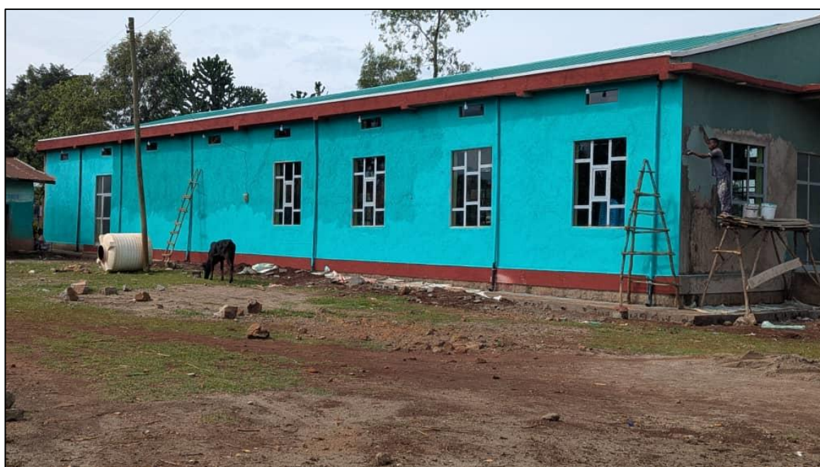
The training hall nearing completion.
